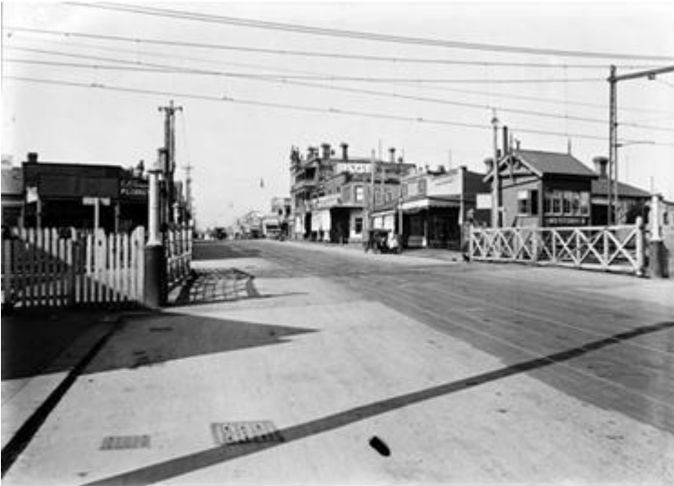
Crossing at St Georges Rd, view north. Public Records Office Victoria, VPRS 12600 P3, ADV/0482
